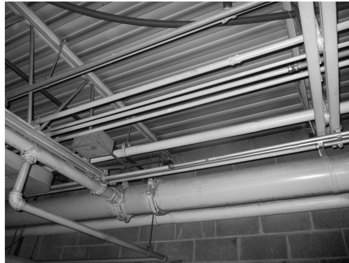
6 MAU-4 STRUCTURAL STEEL INSTALLATION LOCATION NO SCALE
