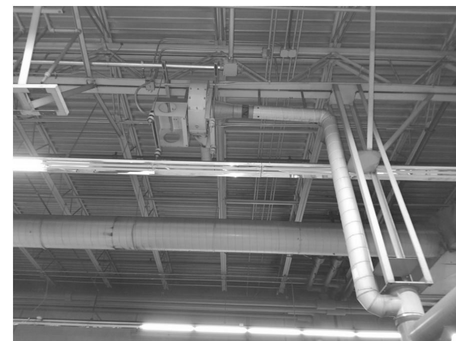
10 ERV-4 STRUCTURAL STEEL INSTALLATION LOCATION NO SCALE
